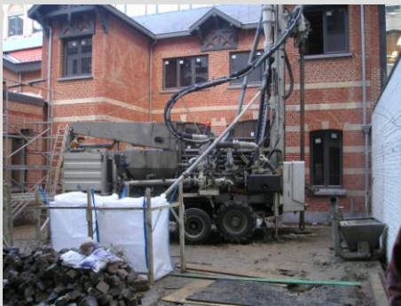
Drilling (2005) and heat pump for geothermal system of REH
