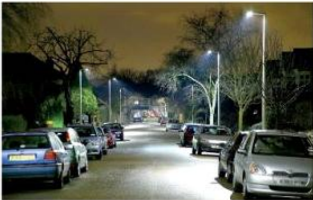
Redbridge, UK, after installation
